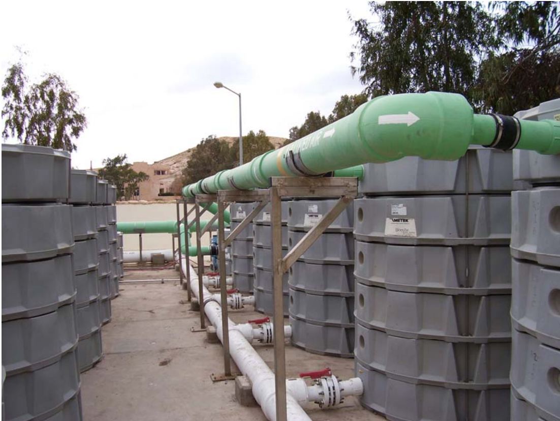
Figure 1: HDPE Modular Biofilters in Parallel (Photo courtesy of BIOREM Technologies Inc.)
