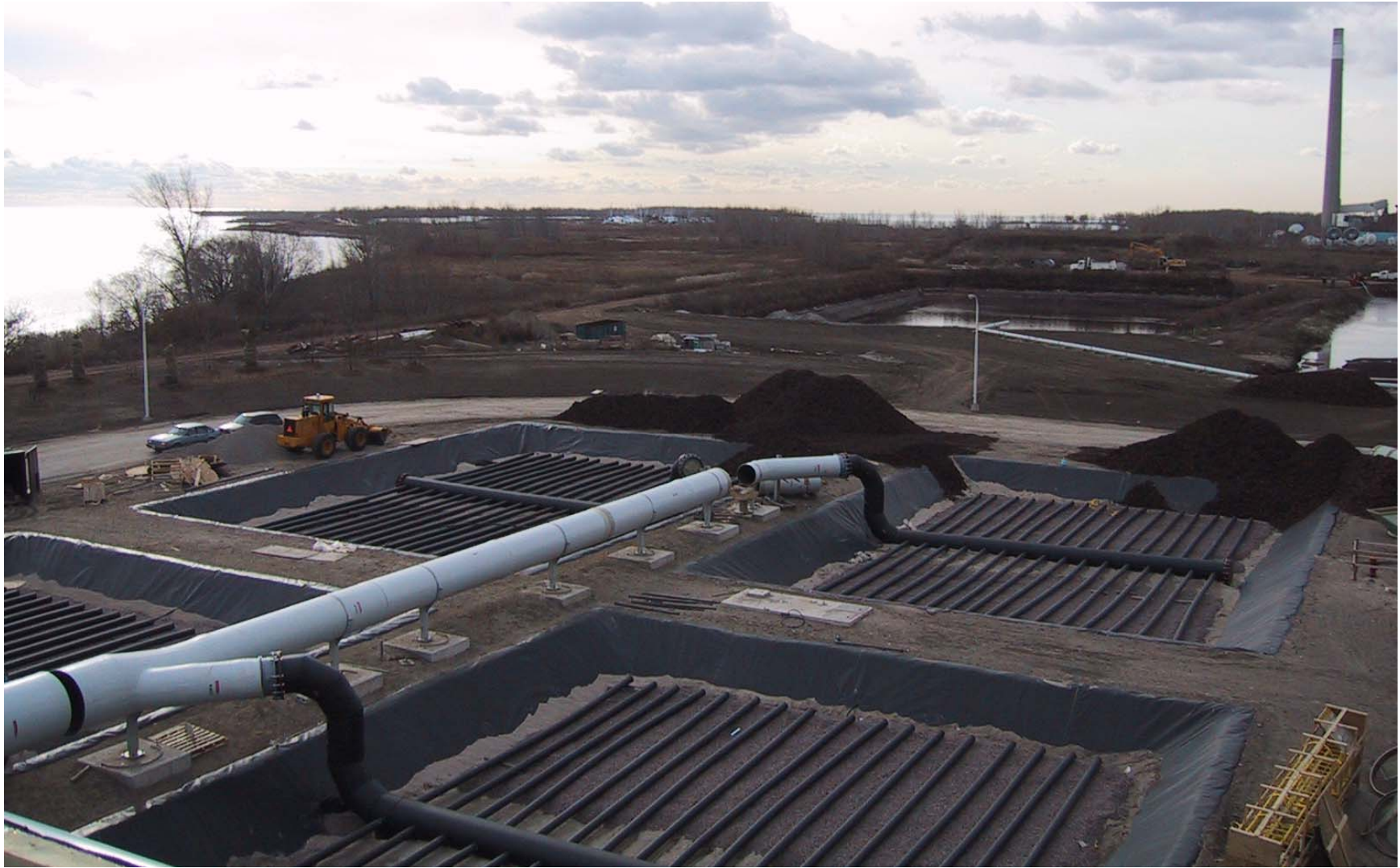
Figure 2: Header/Lateral Biofilter Configuration
